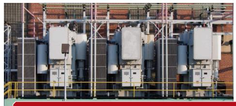
After: Trantech cooling system with seven fans per radiator bank
