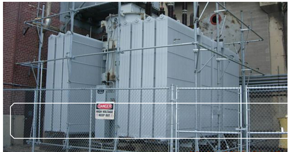
After: Trantech Manifold and Radiator Assembly—no fans or pumps
